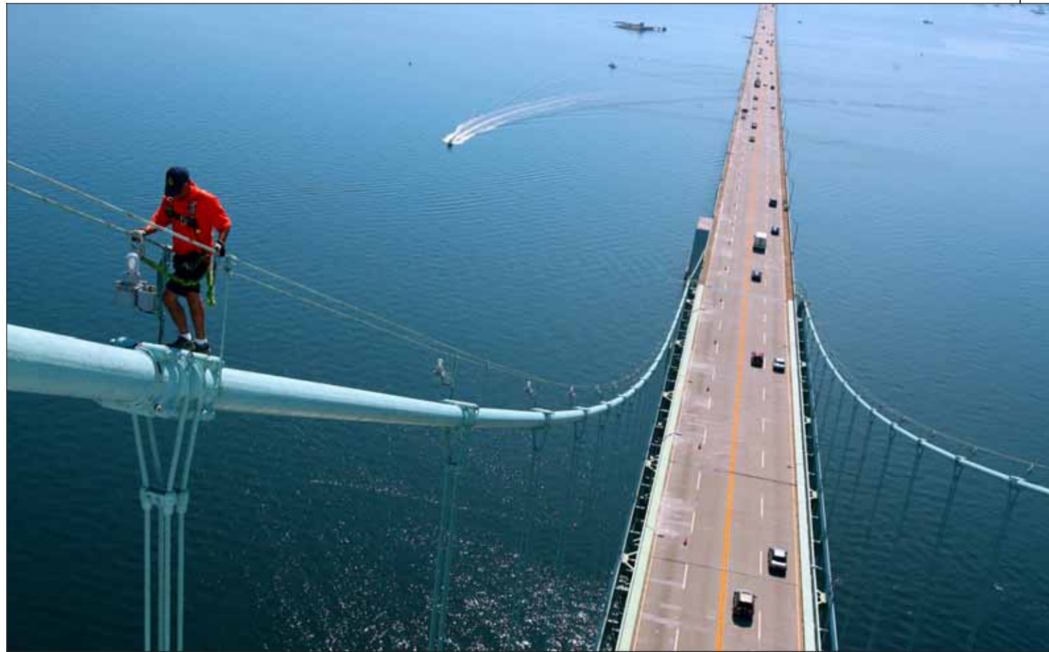
Jim Romano, above, walks the cables of the Claiborne Pell Bridge for various maintenance duties, such as changing light bulbs. Top, engineer Debra L. Moolin-Taylor enjoys the view from the top of the bridge.
